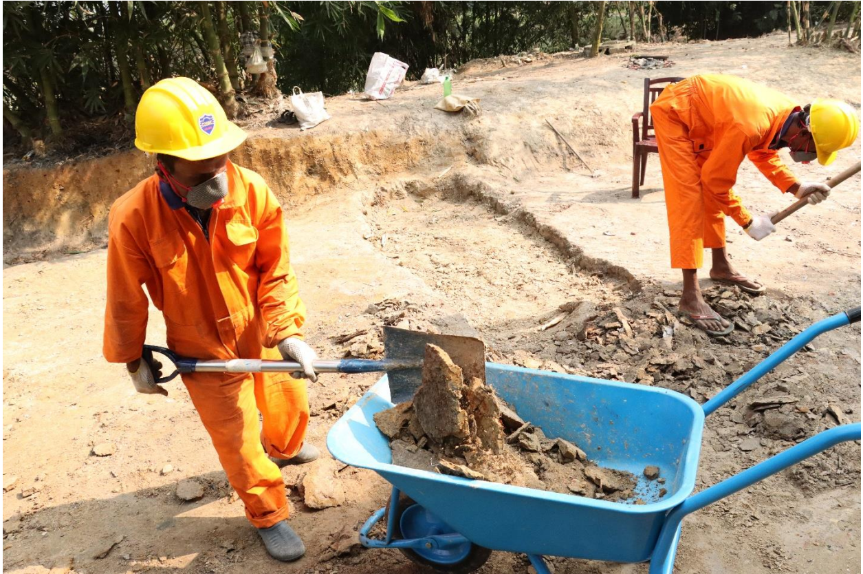
Figure 8. Workers removing surface layer of contaminated soil.
