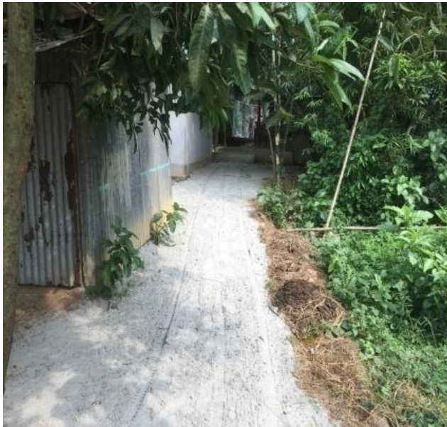
Figure 9. Spreading of clean soil in scraped house yards.
